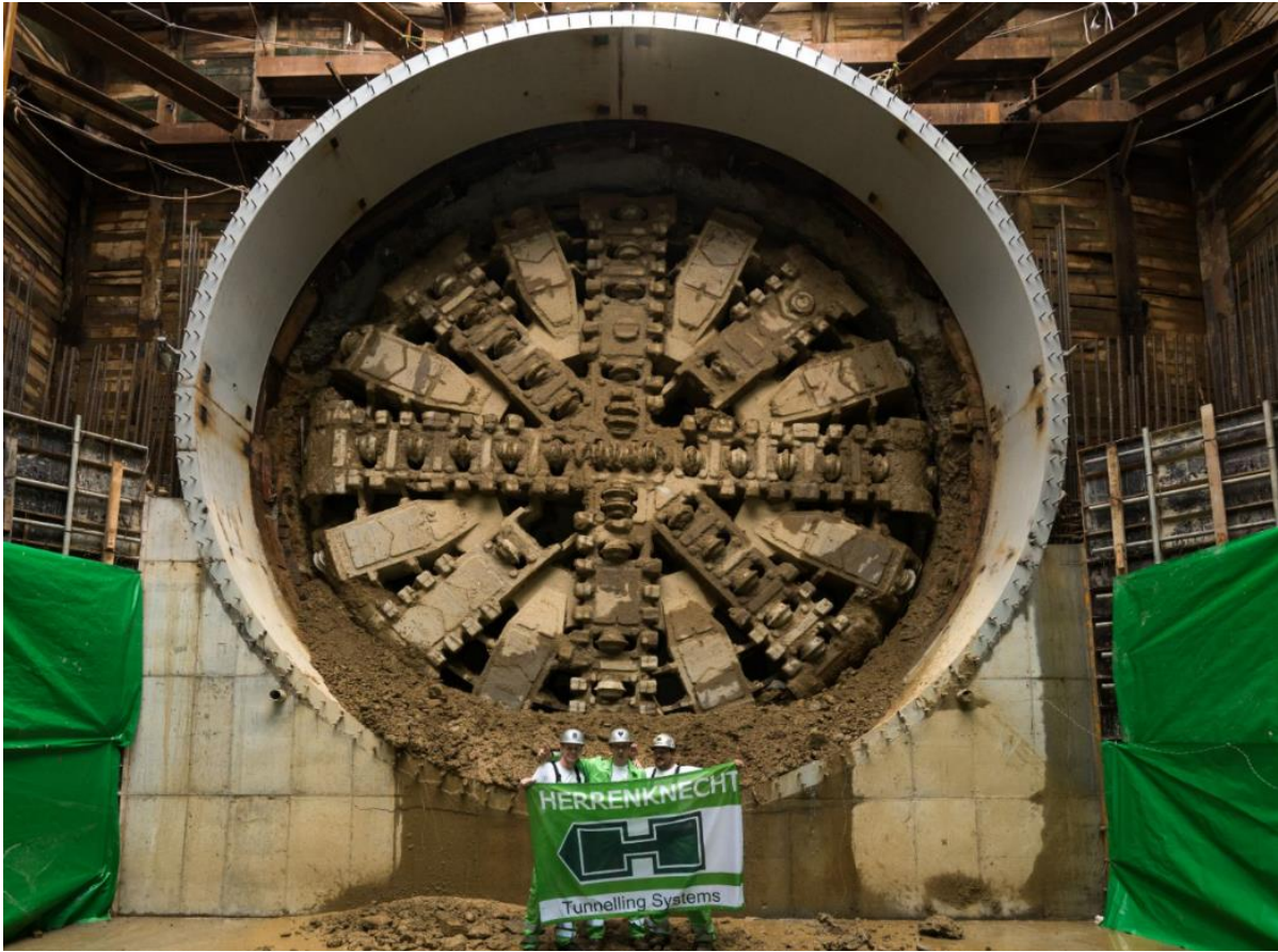
Fig. 11 Successful TBM break-through of the project.
