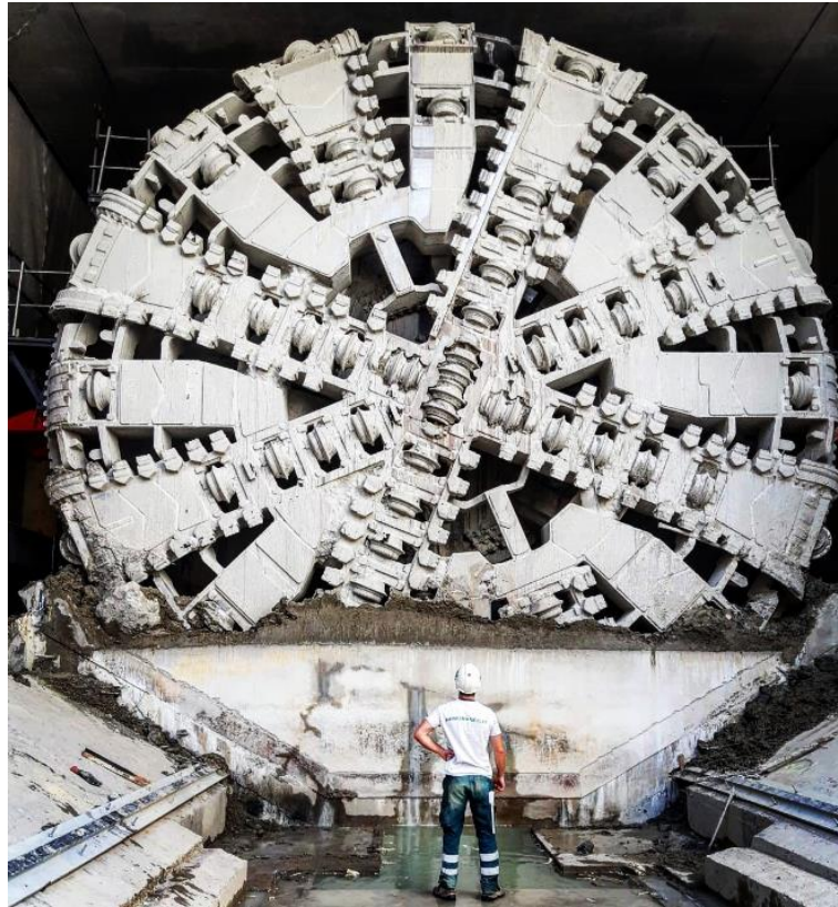
Fig. 18 Successful TBM break-through of the project.
